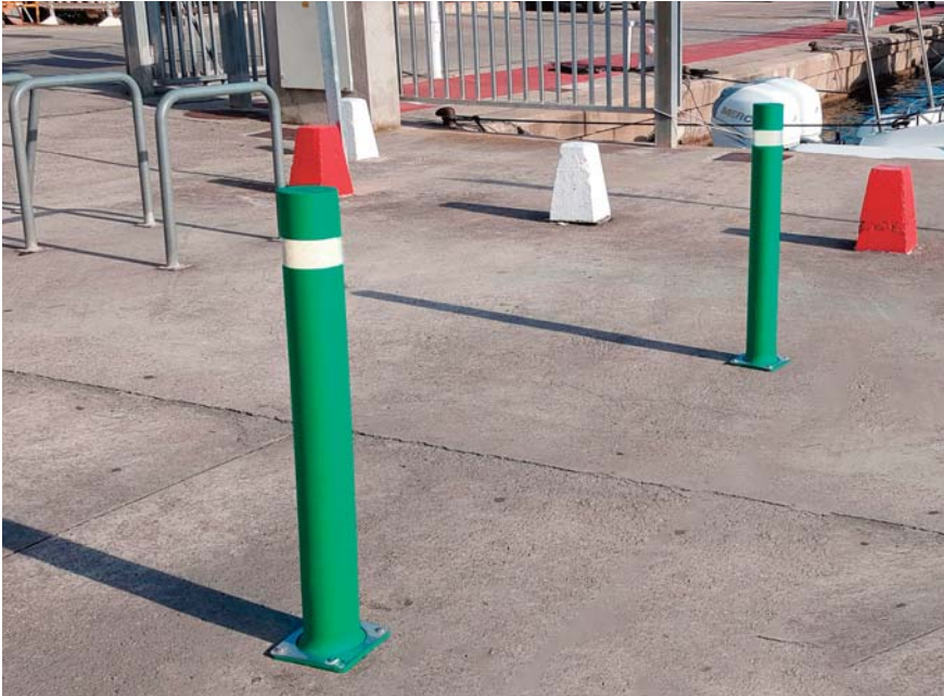
Detail base with a reinforcing plate for a major fixing to the ground.
